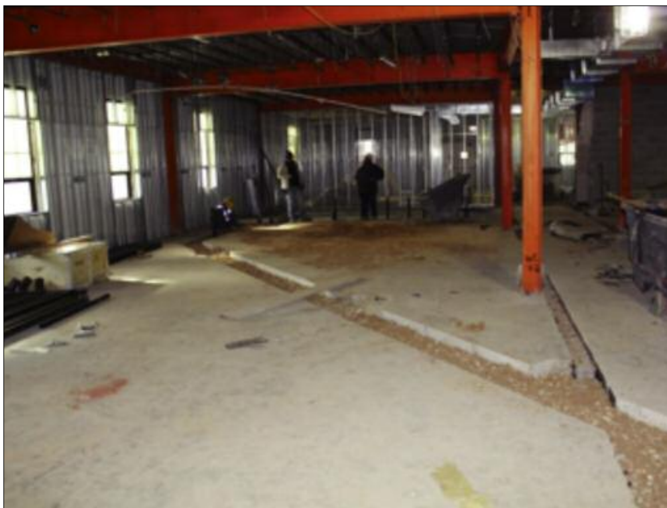
Renovation of Building 1442 — Photo: Staff
