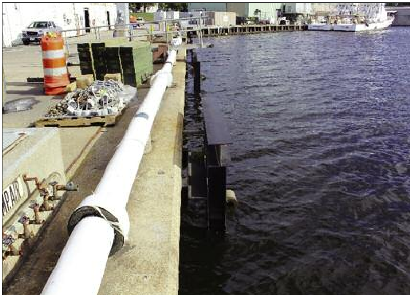
Repair and Wharf Fendering System, Baltimore, MD — Photo: Staff
